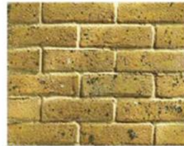
Yellow London stock brickwork
