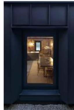
'Greencoat PLX' metal cladding
